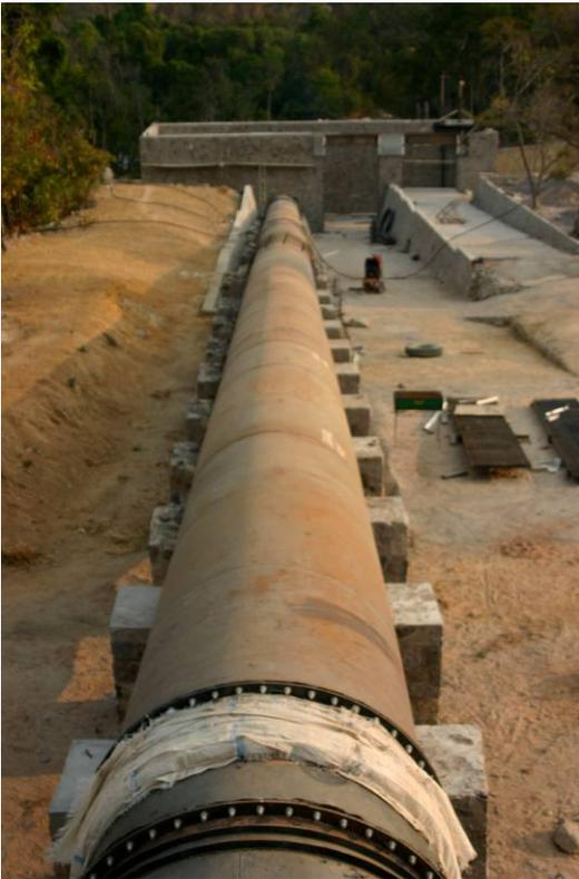
The penstock pipe to deliver water to the turbine
