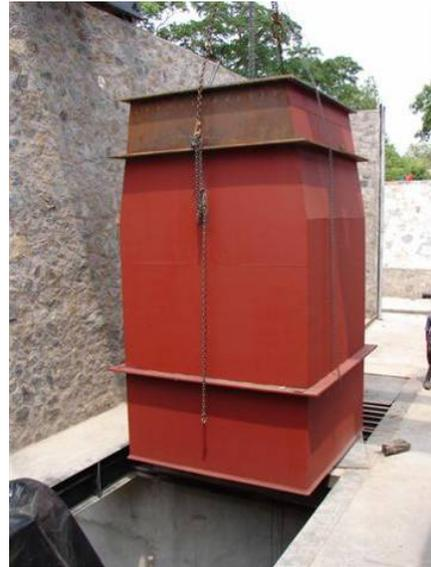
**The Draft Tube into the sump structure under the power house**
