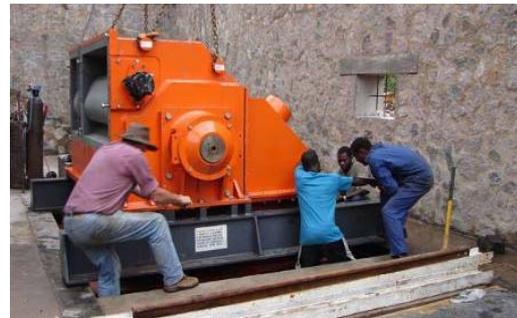
**Connecting the Turbine to the Draft Tube on the floor of the power house**
