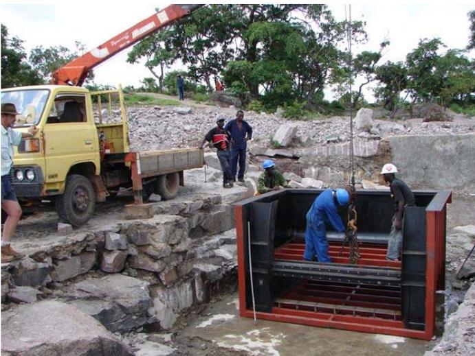
The sediment chamber Sluice Gate installed
