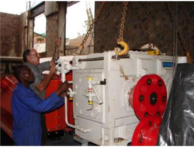
The Gearbox lowered into position next to the turbine (behind)
